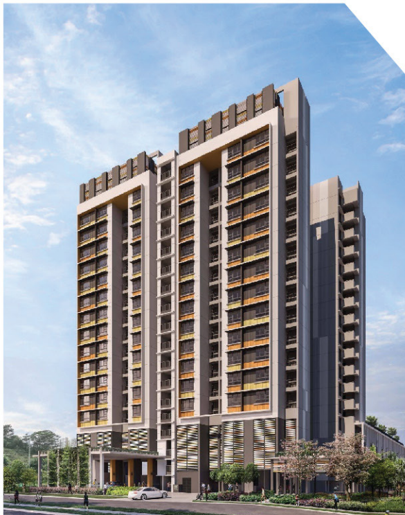
HDB Community Care Apartment
